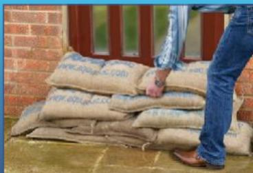
Remove any debris from the area. Drop the bags into place to help eliminate gaps and create a seal (interleave a plastic sheet between layers of bags to improve the seal). Place bags in layers, like courses of bricks in a wall.
